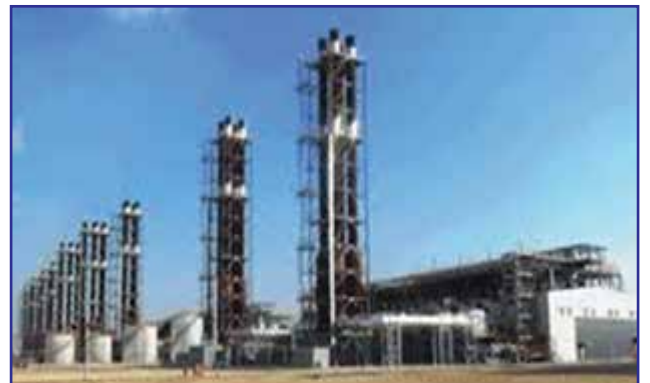
JORDAN IPP3 POWER PLANT
