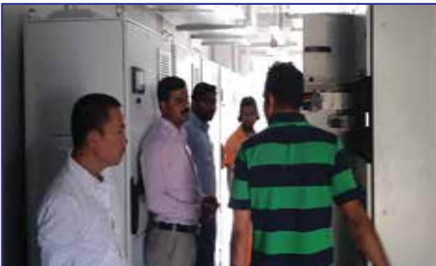
FACTORY ACCEPTANCE TEST
